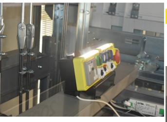
The **GMS375** incorporates two bright LED strip lights molded into the top of the inspection box.
